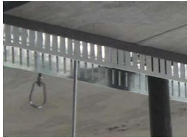
Fig. 5 ClarkDietrich BlazeFrame deflection track with factory applied intumescent tape
